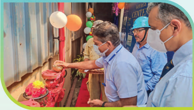
Installation of Water Sprinkle System in DA Supply Room of PP Shop, Main Unit on 16 Aug 22
