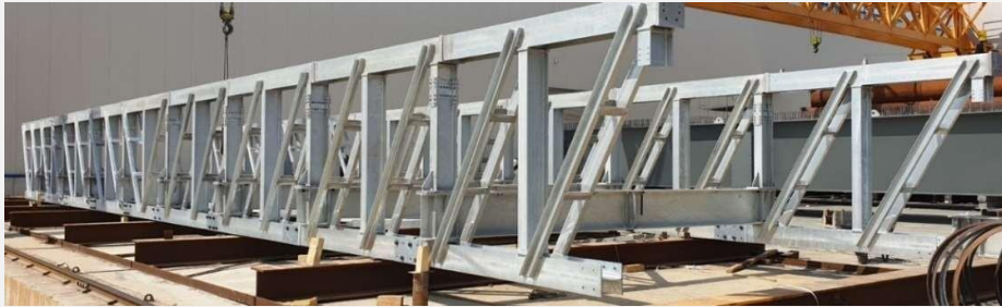
Fig. 4 - Validation geometric control Modular Bridges
