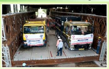
GRSE make "Double Lane Portable Steel Bridge", the pre-fabricated bridge has a span of 42.67m without intermediate pier and a width of 7.5m. It can support two-way traffic comprising heavy vehicles with a total load of about 110MT. With a modular design facilitating easy assembly, these bridges can be erected quickly even in the most demanding terrains and conditions.
